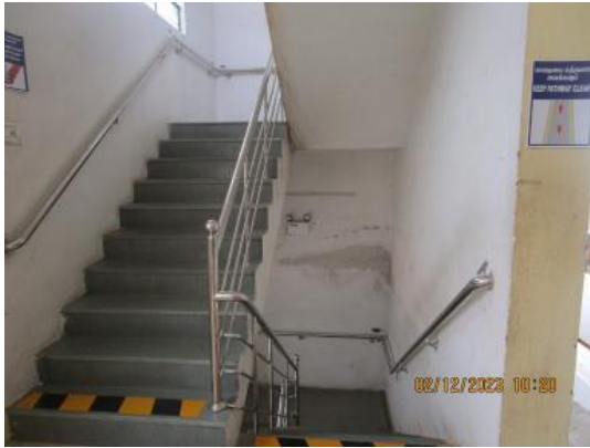
Emergency exit stairway.JPG
