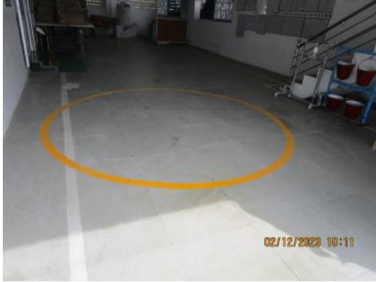
Safe assembly point.JPG
